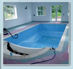
This Rectangle Hopper pool with roman end steps was originally an outdoor pool which was refurbished to become an indoor pool with suitable equipment added for disability access. The pool was first fitted with new underlay. Then a blue mosaic patterned liner was hung and a vacuum placed in order to set the liner air tight to the underlay. The vacuuming process helps to eliminate any creases to achieve a smooth finish.
