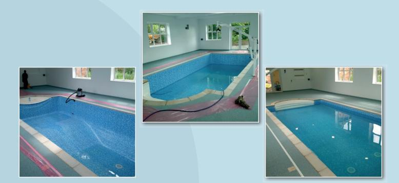
The pool is now ready to be filled half way with fresh water ready for the pool fittings to be put into place. The vacuum can be removed and the pool is now filled to the correct level. The resin rubber chipped flooring is laid in order to minimise any slip hazards.
