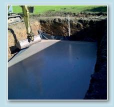
The chosen size and shape of your pool has now been determined so the journey begins. Preparation of the ground starts and the hole will be dug to the size and depth of your pool. A digger is usually required for this. Once the ground has been dug out, a concrete slab is then poured in.
