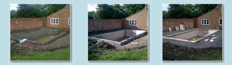
The area around your pool is back filled and the walls are now built and rendered with concrete.
